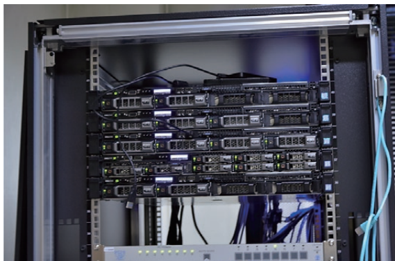
演習室用サーバ Servers for Seminar Rooms
