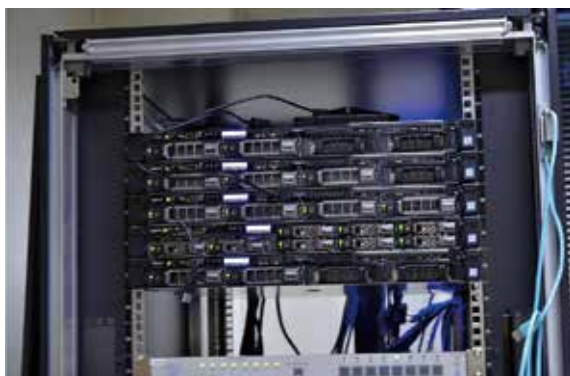
演習室用サーバ Servers for Seminar Rooms
